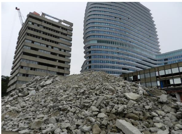
Figure 2, Demolition of concrete
